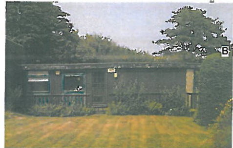
VIEW OF EXISTING CHALET FROM MAIN HOUSE
